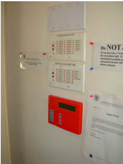
11. Fire detection - monitoring panels
