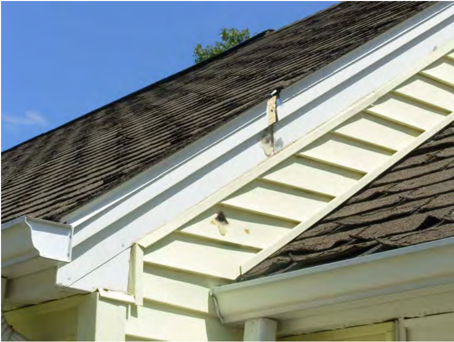
5. Spot trim and vinyl siding damage
