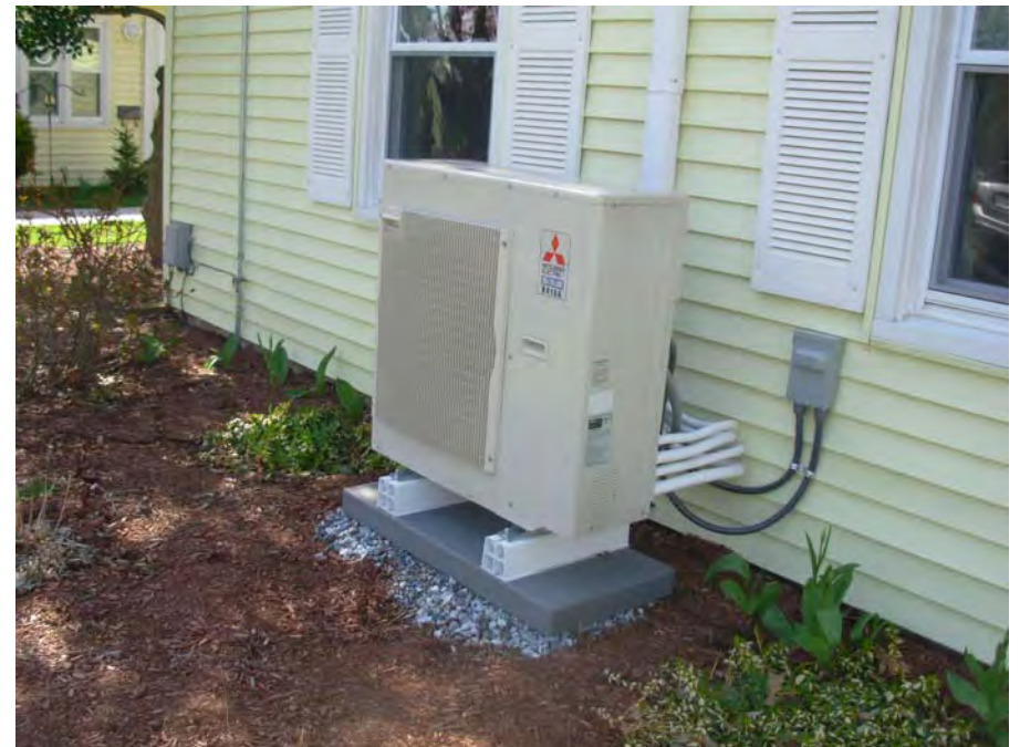
12. Typical heat pump HVAC system exterior condensers
