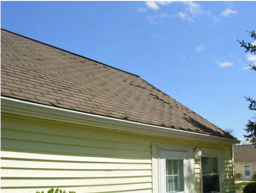
7. Lifting and curling of roofing shingles
