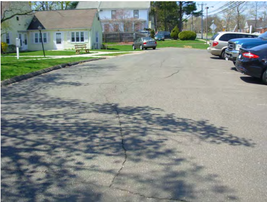
1. Sporadic cracking of parking paving
