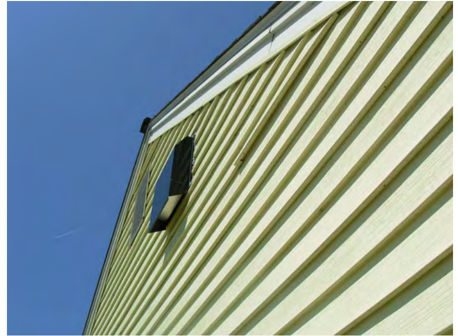
6. Spot seam popping of vinyl siding
